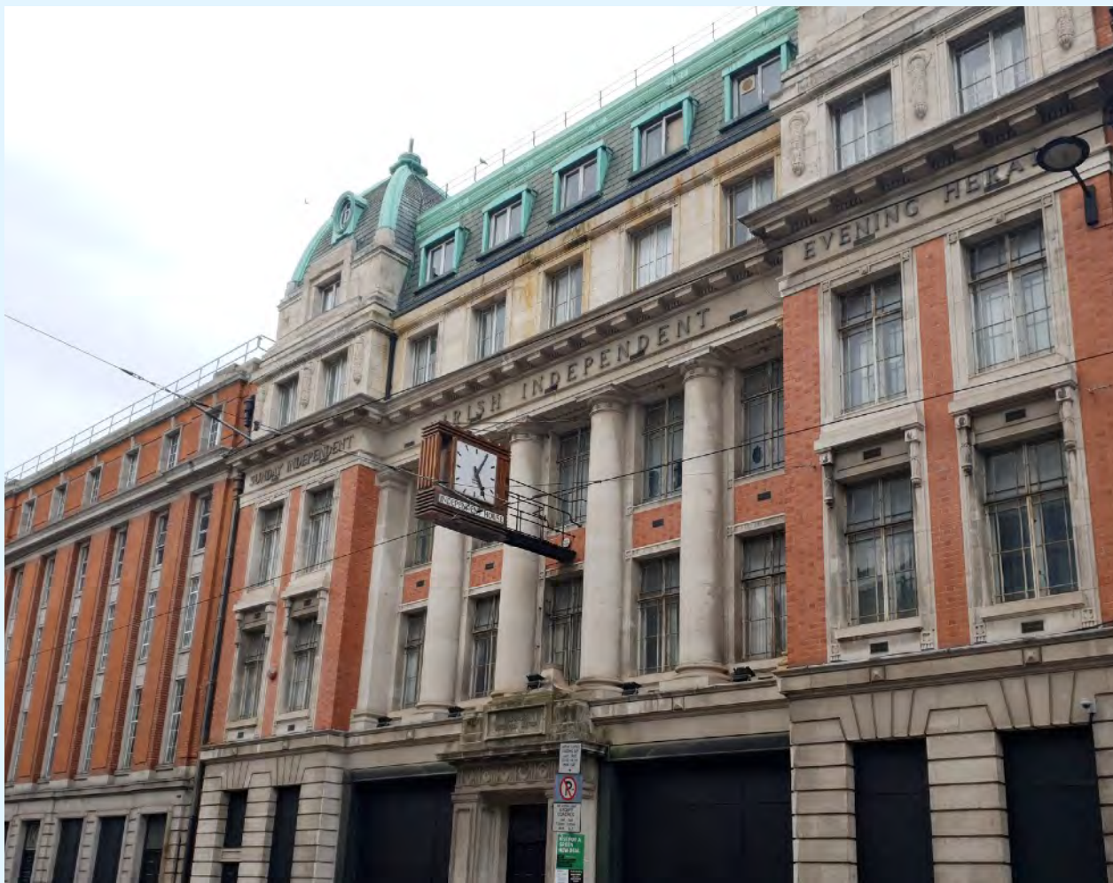
Independent House on Middle Abbey Street, constructed in 1924 and home to the Irish Independent until 2004, when Independent News and Media moved to Talbot Street. The copper-framed clock in the centre of the façade – “Set your watch by it”, as the line used to go – appears to have stopped in the years since.
